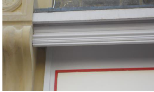
Cornice incorporating recessed lighting
