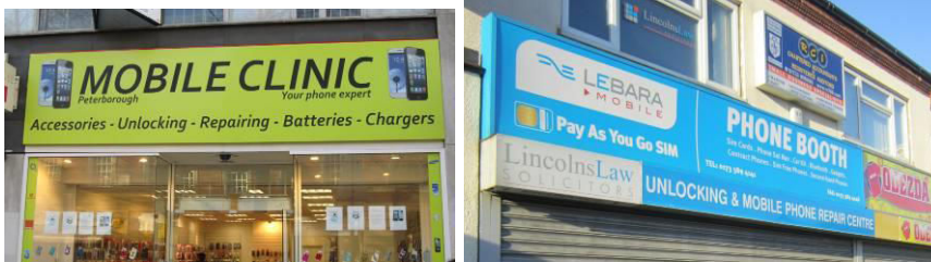
Inappropriate oversized fascias and deep projecting box fascias
